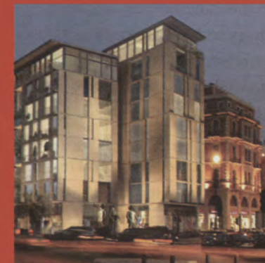
Foch 94 residential development, Lebanon
